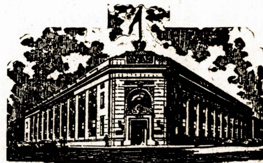
STANDARD FEDERAL BUILDING
