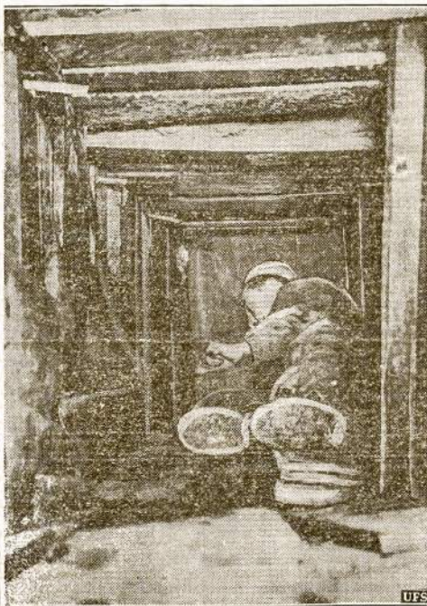
JOB WAS FUTILE - Hole 50 feet long was tunneled under Cherry Hill prison cells, at Philadelphia, by convicts seeking to escape. Prison officials discovered it. Jan. 15 Wilson of Williamsport, convict leader, was reported suicide.
