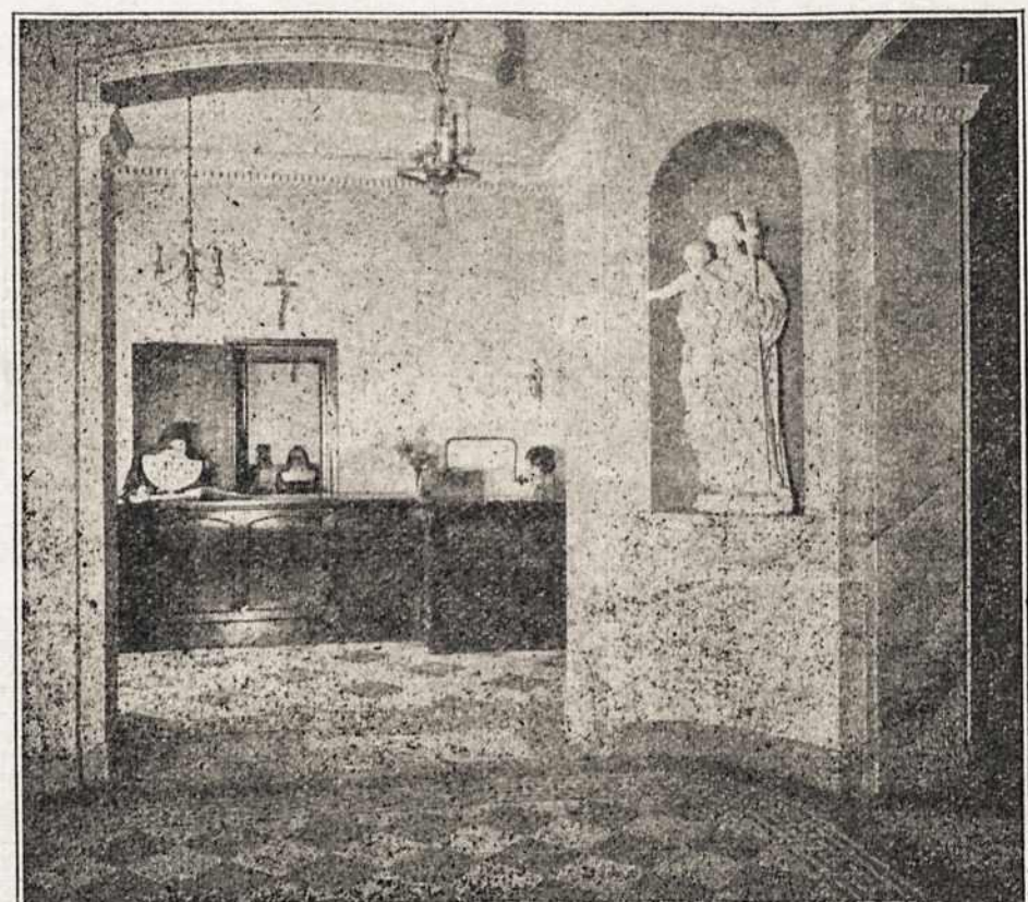
LOBBY AND OFFICE
