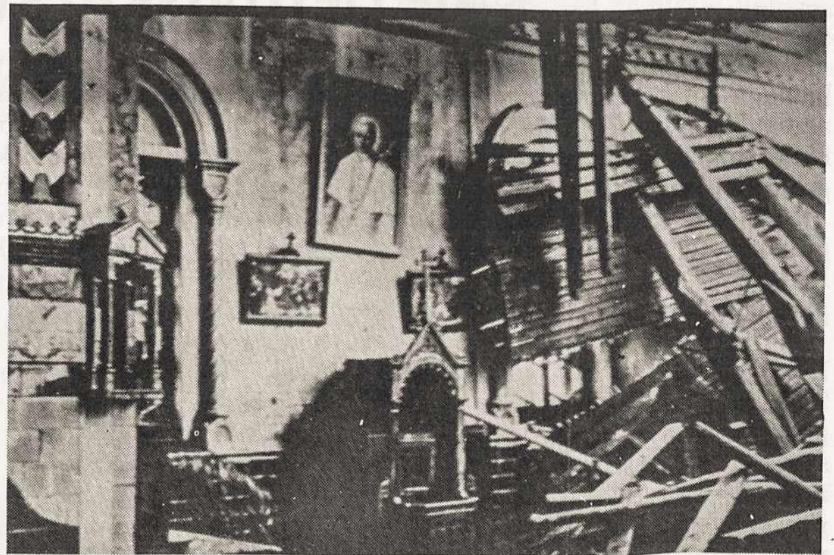
St. George Church, Šiauliai, Lithuania left — exterior, before "mysterious" burning, above — interior, after fire, where firemen stood by and watched.
